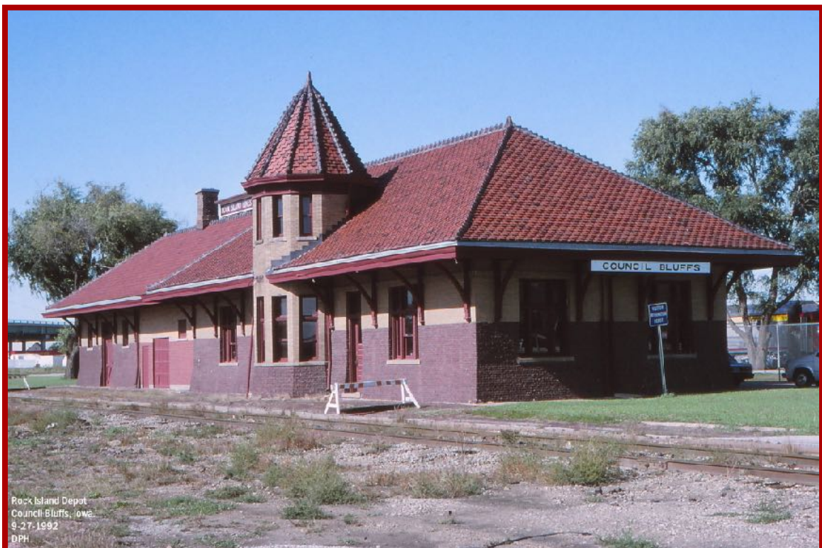
Below: RI Depot @ Council Bluffs, Iowa 9-27-1992
